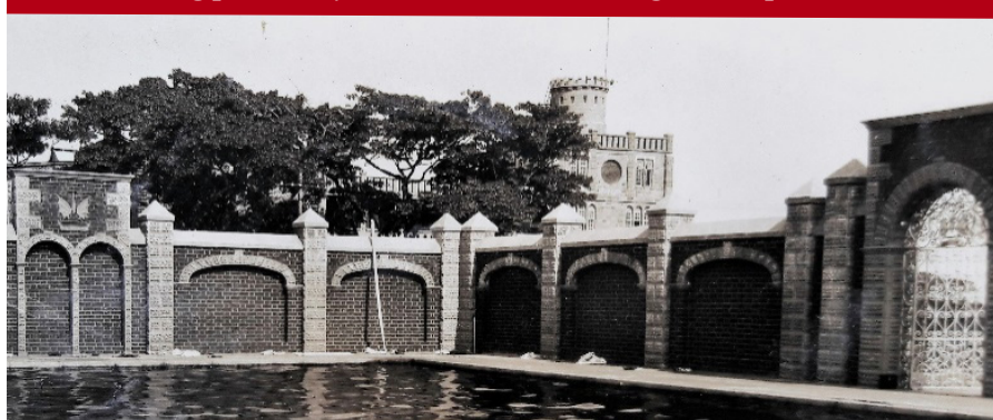
Old swimming pool, early 1930s, with decorative gate and perimeter wall.
