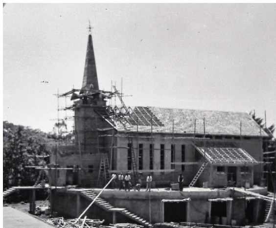
Hartmann House Chapel under construction, late 1957.
